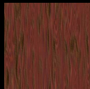
Rotten Red Wood
